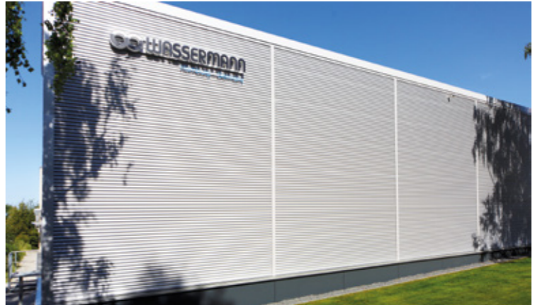
High rack storage area
